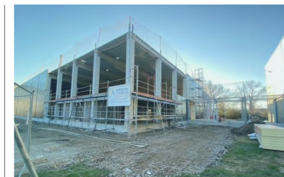
The new logistics hall in Ahlen is taking shape.
