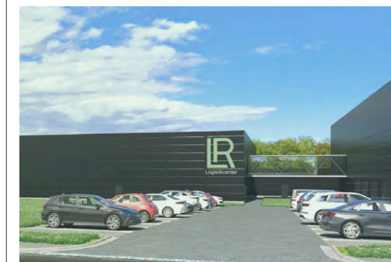
This is what the new logistics hall in Ahlen will look like in the future.
